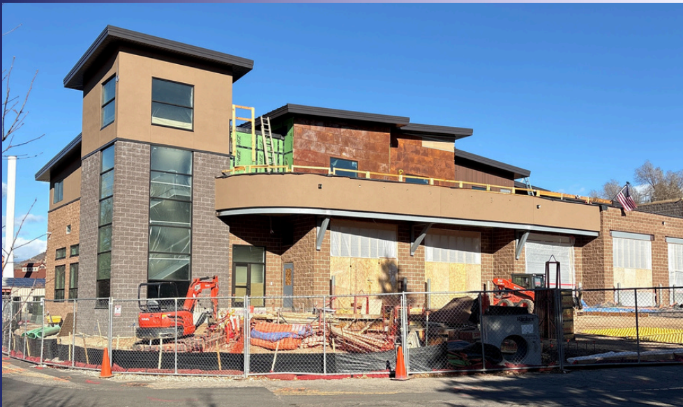
Station 2 - Under Construction
